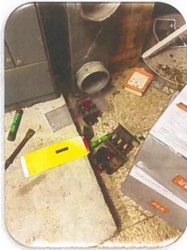
Figure 31 Broken Circuit Breakers in Control Room
