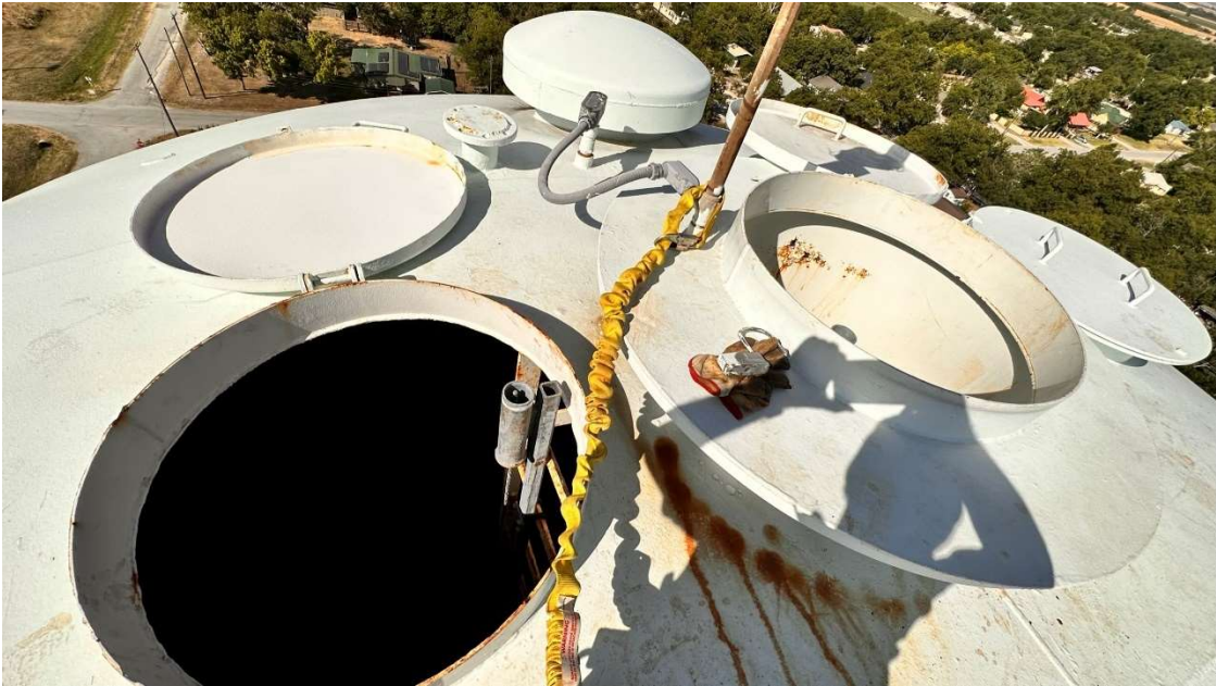
Photo #8: Top of Tank
